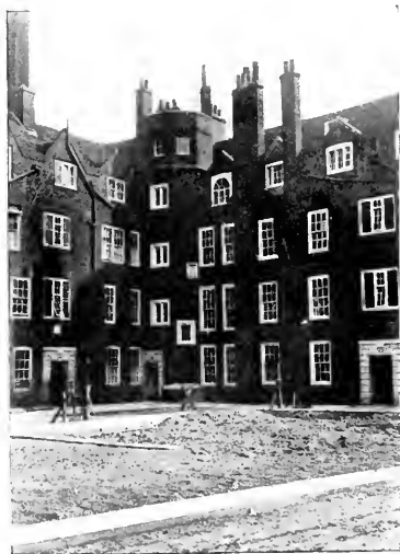
121. Old Buildings, Lincoln's Inn.
